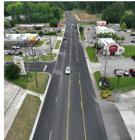
North Chalkville Road improvements and resurfacing completed during 2025
