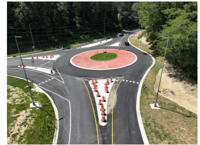
Opening of the new roundabout at Sicard Hollow Road that removed a dangerous intersection and improved it with a roundabout configuration that is safer, and keeps traffic moving
